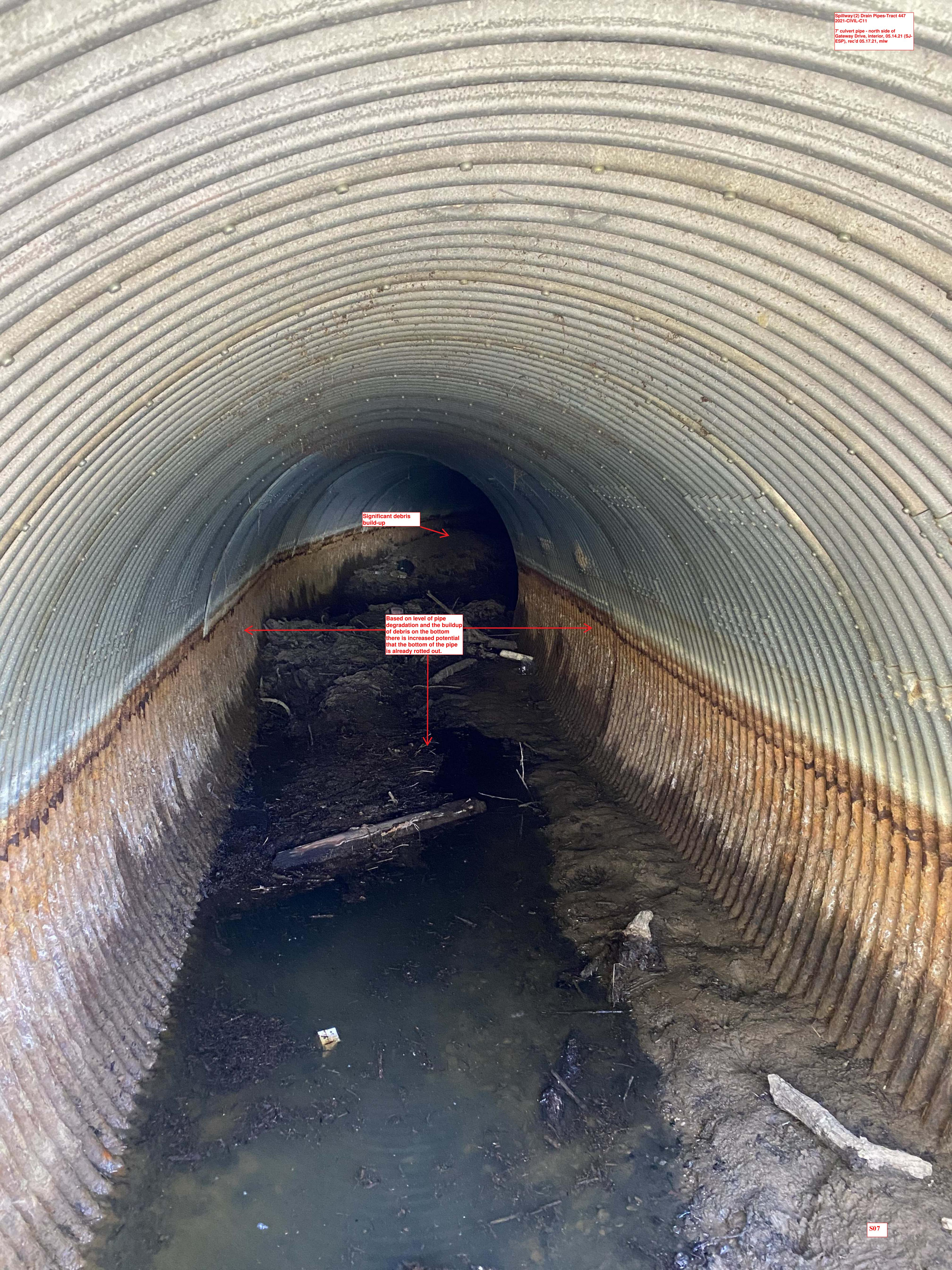
Significant hole under pipe.
