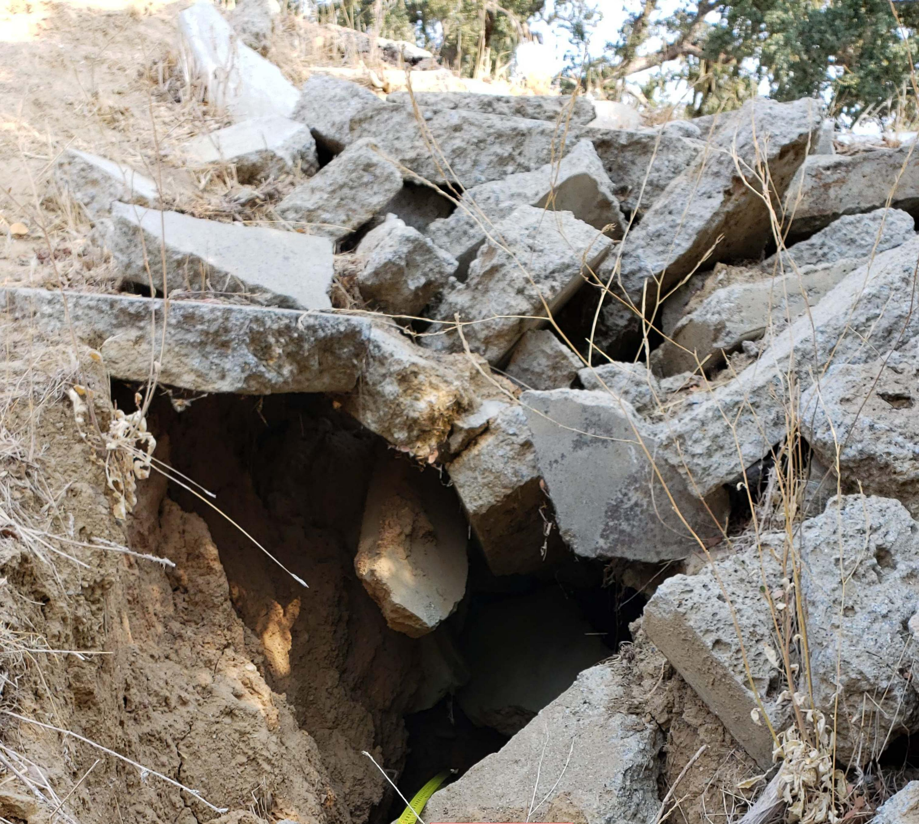
From the face of where the rock is supposed to be there is a 7' plus void which goes back past the 2' hole towards the road edge.
