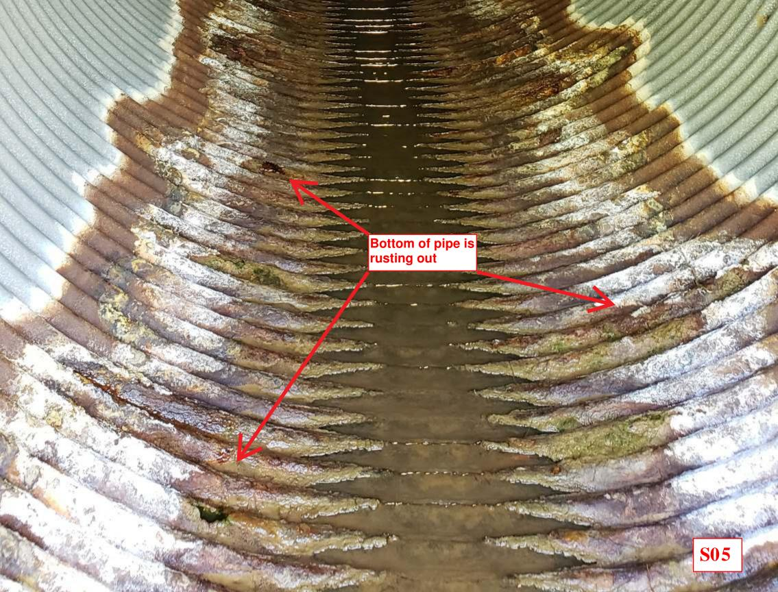
Bottom of pipe is completely rusting out.
