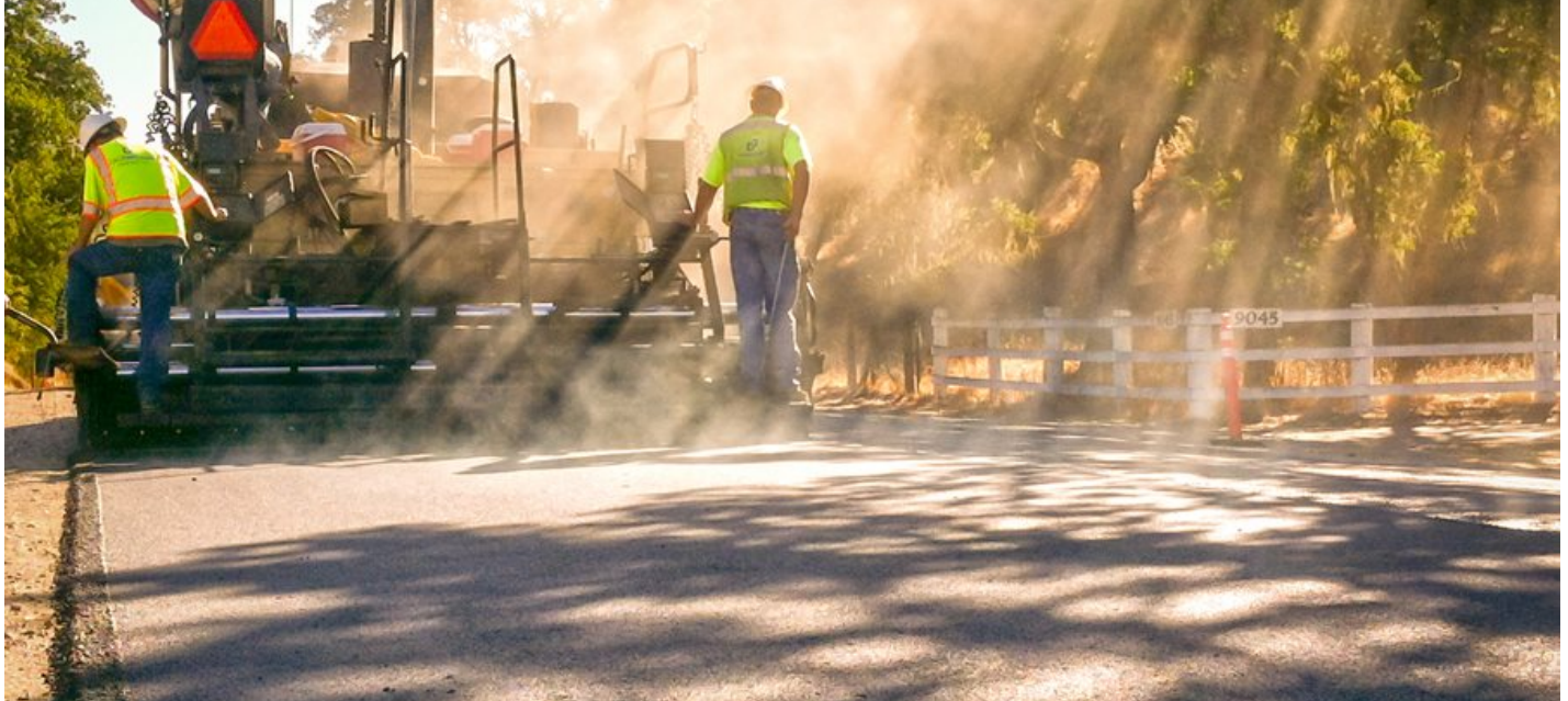
Asphalt Overlay North County Roads
