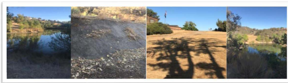
View from south side crossing dam to N. side Bluebird Lane access view from north side
